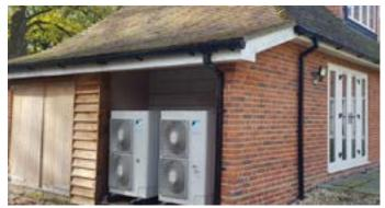
Figure 59: Place pumps in a recessed space to minimise the visual impact
